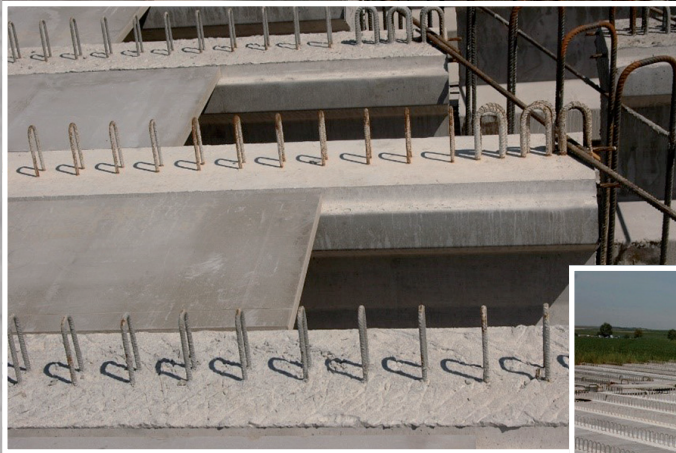
BETONYP® as formwork
