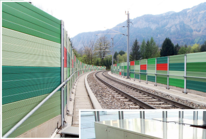
BETONYP® as noise reduction wall
